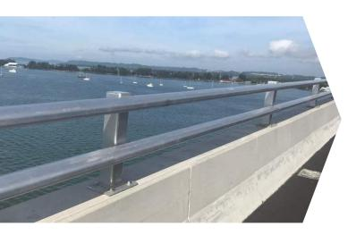
VarleyGuard and V6Guard bridge parapets are compliant with the European EN1317 standards whilst VGAN 300 and VGAN 400 meet American standards NCHRP350 and MASH respectively.
