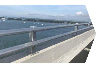
VarleyGuard and V6Guard bridge parapets are compliant with the European (EN1317) and American standards (NCHRP350 and MASH).
